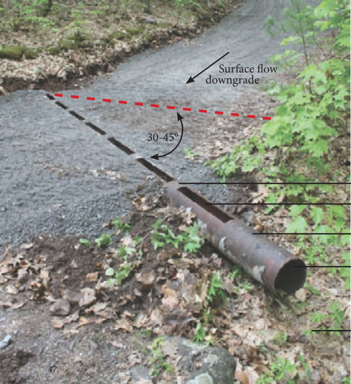
PHOTO 2: OPEN TOP PIPE CULVERT
