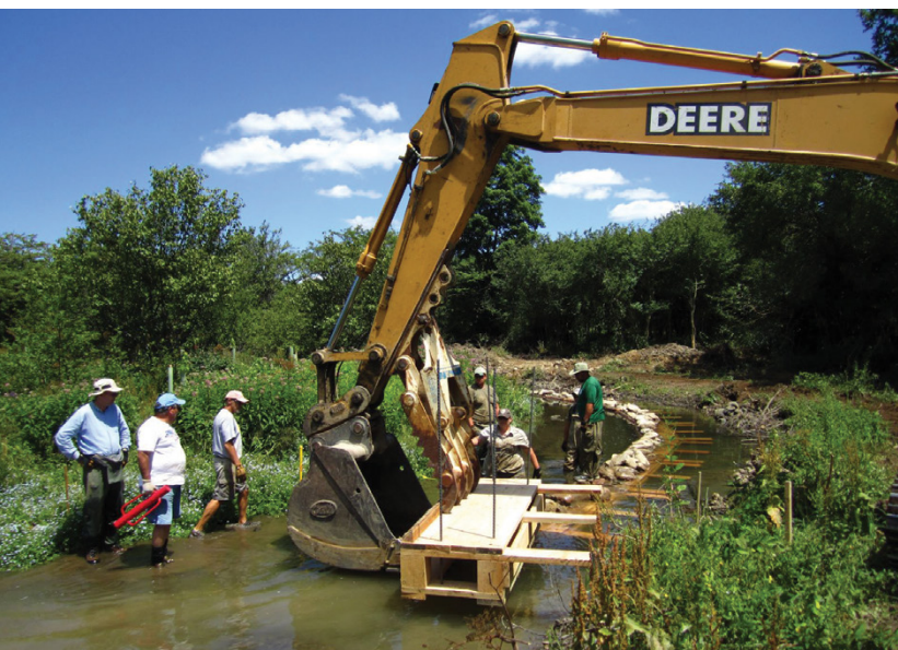
Installing lunker structures
