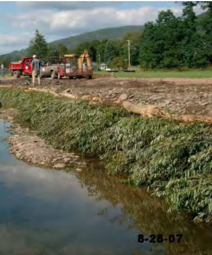
LIVE CRIBWALL (Not to scale)
