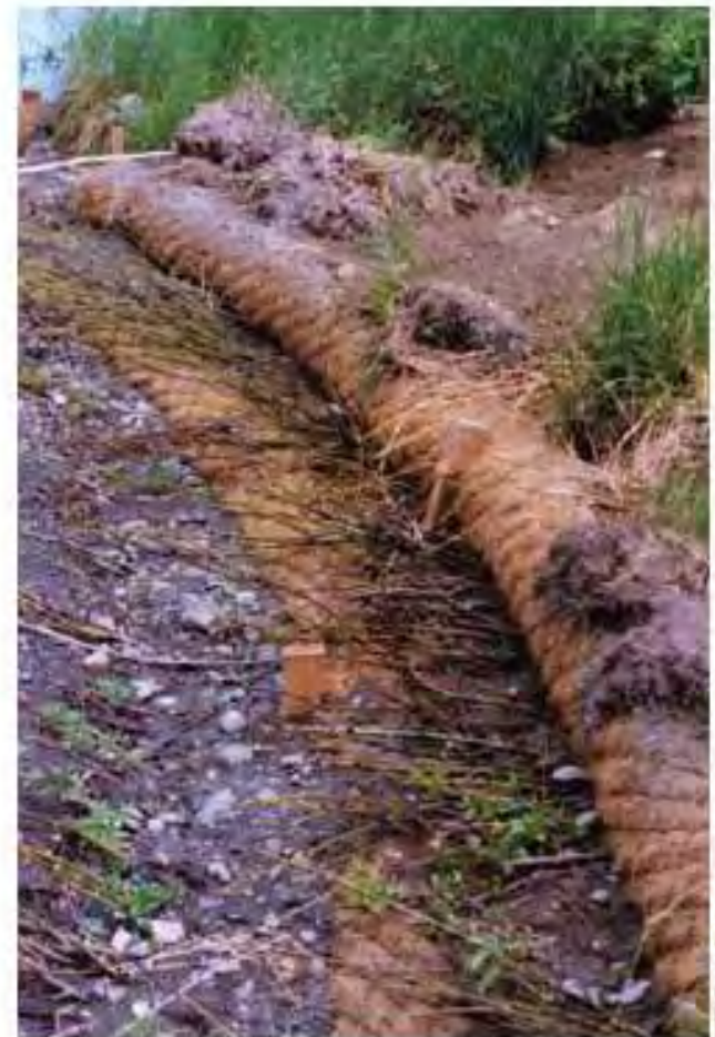
Brush layering with coconut logs.
