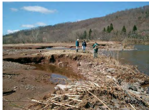
Figure 3.12 Berm that was breached in 2005 storm event
