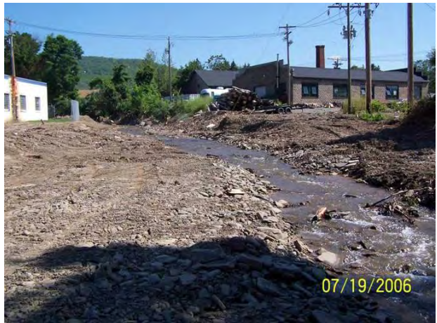
Figure 3.14 Stream channel after Post Flood Intervention.
