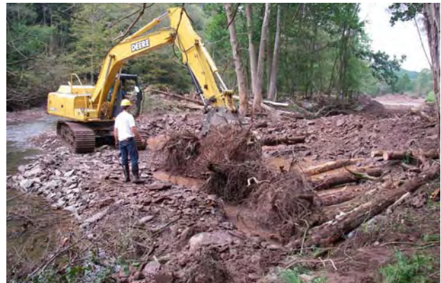
Figure 3.16 Root wads were placed in two layers with large boulders or logs to hold them in place
