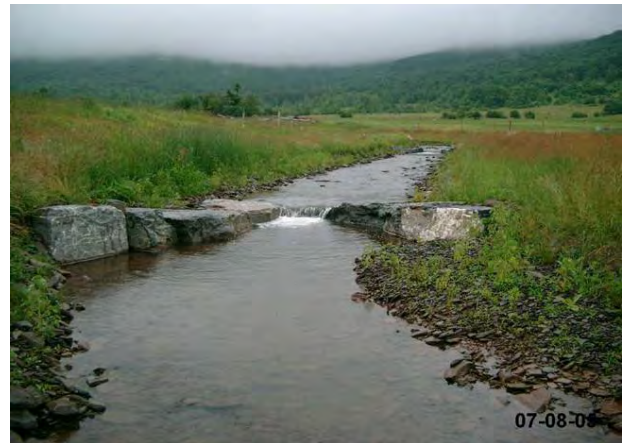
Figure 3.19 Rock Cross-Vane
