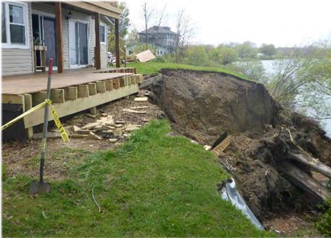
Figure A.4-4. Bluff erosion and collapse along the shoreline of Lake Ontario. Development sited close to the crest or edge of a bluff can be more vulnerable to collapse, especially in strong storms.
