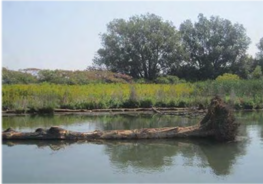
Figure 3-10. Lagoon of Strawberry Island in the Niagara River. Tree trunk and rootwad installed and anchored in water to act as a low-profile sill that will attenuate waves and currents. Vegetation has become established behind the tree along the shoreline.
