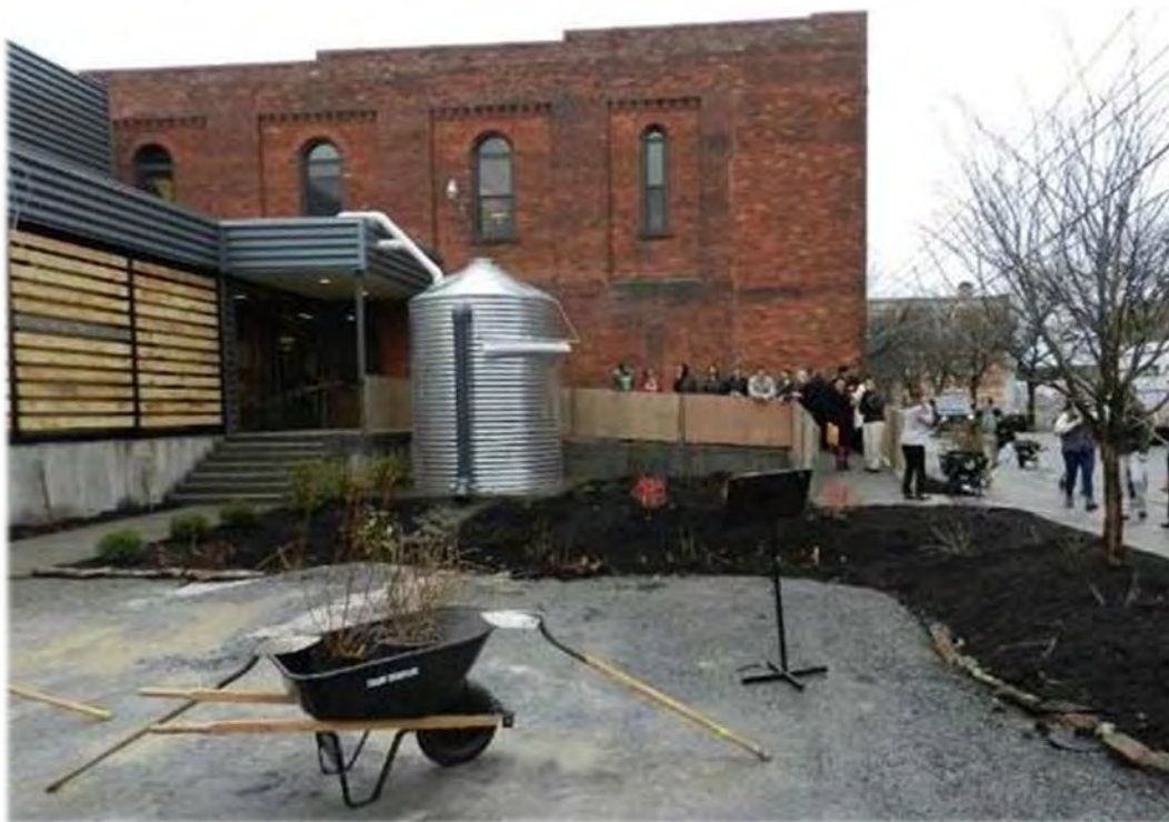
Figure A.18-2. Cistern collecting rooftop runoff and diverting it to a rain garden in Troy, NY.
