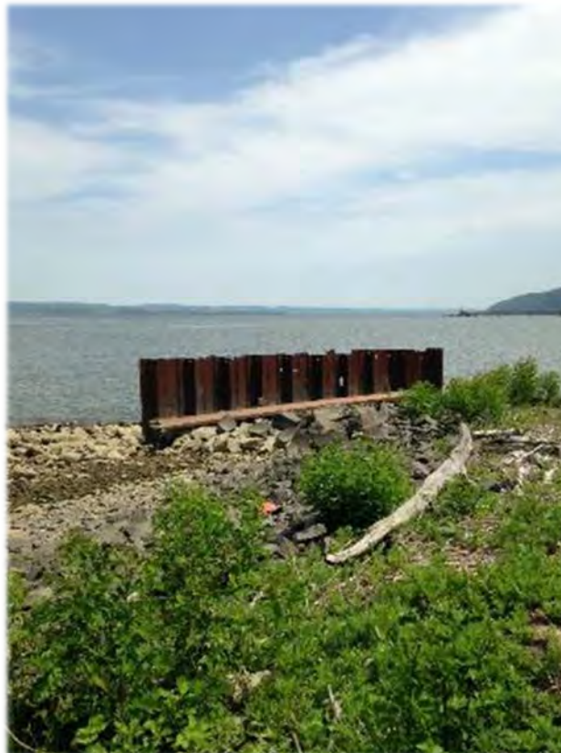
Figure D-2. Steel cap of sheet pile bulkhead at Haverstraw Bay Park on the Hudson River that was dislocated by Hurricane Sandy. Such damage could require significant repair and replacement costs.
