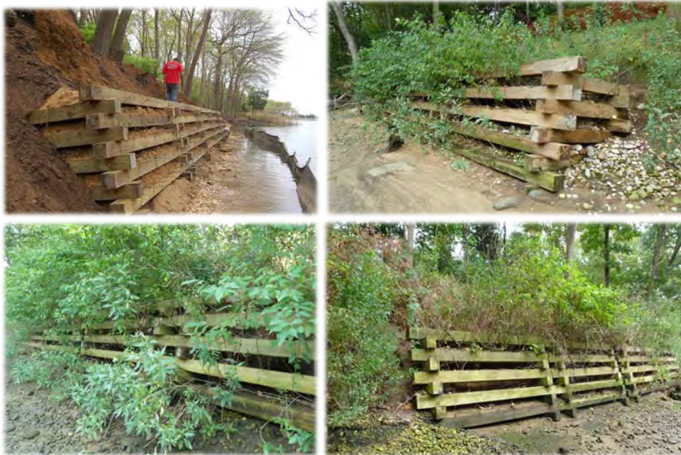
Figure A.19-4. Live crib wall monitored for five years at Stony Brook Harbor, NY. Upper left: installed in 2009; upper right: one year later; lower left: three years later; lower right: five years later.
