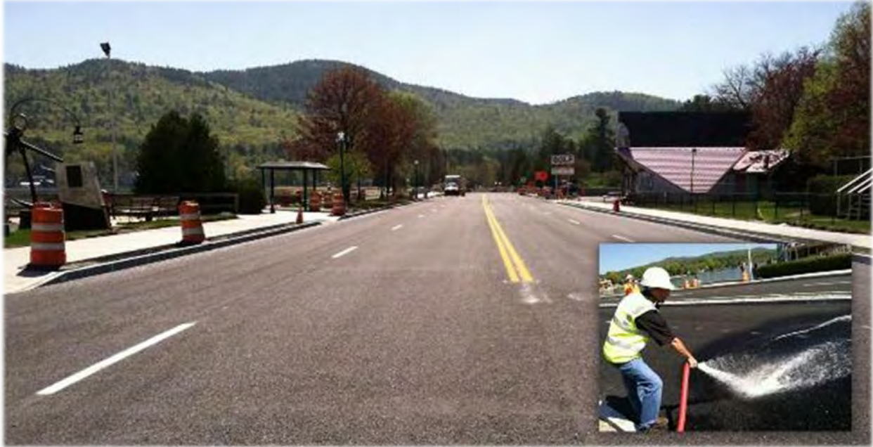
Figure A.18-6. Porous pavement and a demonstration of infiltration in Lake George, NY.
