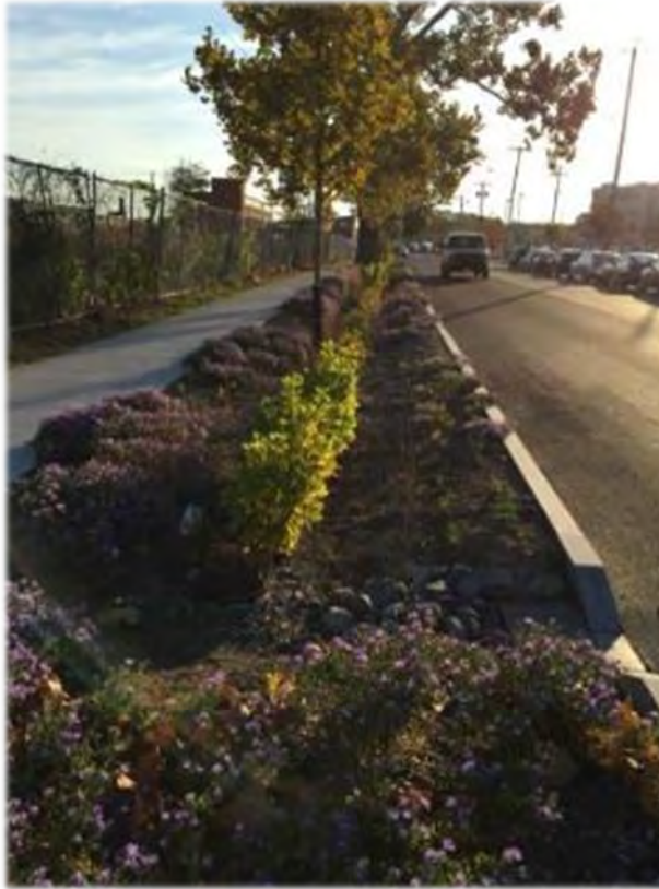
Figure A.18-1. Bioretention area capturing runoff from street in Syracuse, NY.
