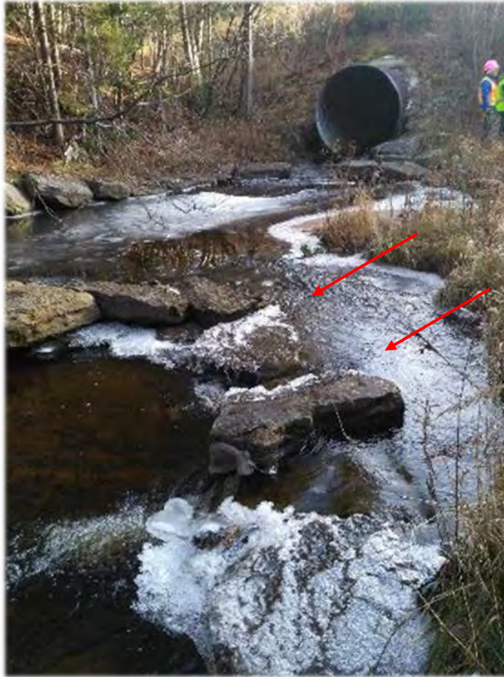
Figure A.20-5. Use of a rock vane to redirect water flow from a culvert and reduce erosion on the streambank. Red arrow points to the rocks in the vane. Flow from the culvert is being directed by the vane to the right and then back to the left over the rock vane.
