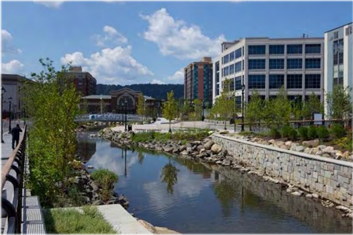
Figure A.20-8. Daylighted Saw Mill River in Yonkers, NY. Prior to this project the stream ran underground beneath parking lots in a business district.
